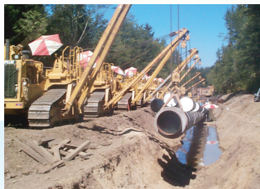
Inspection and repair of coating
