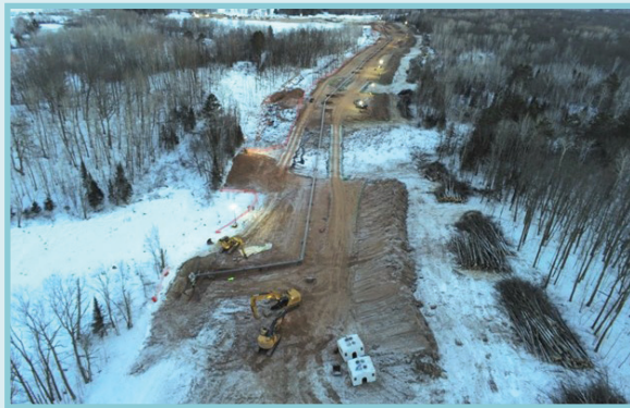
Temporary Bypass Line Installed Around Rupture.
