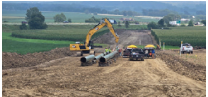
M530B Pipeline Replacement - 26-inch diameter pipe.
