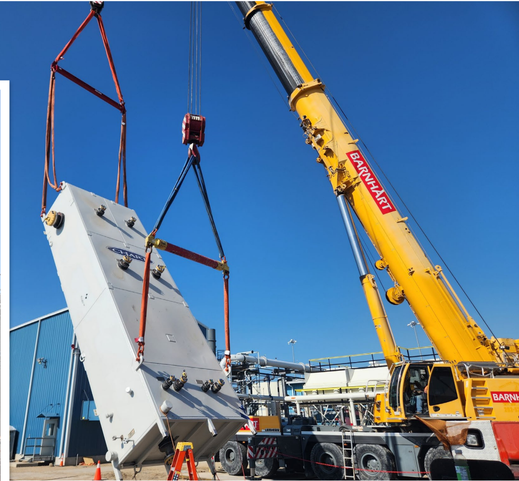
2024 cold box installation at the Garner LNG facility
