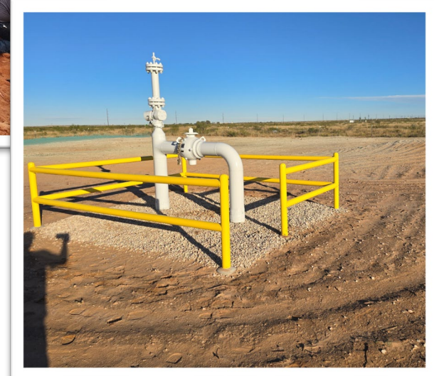
10-inch tee replacement
