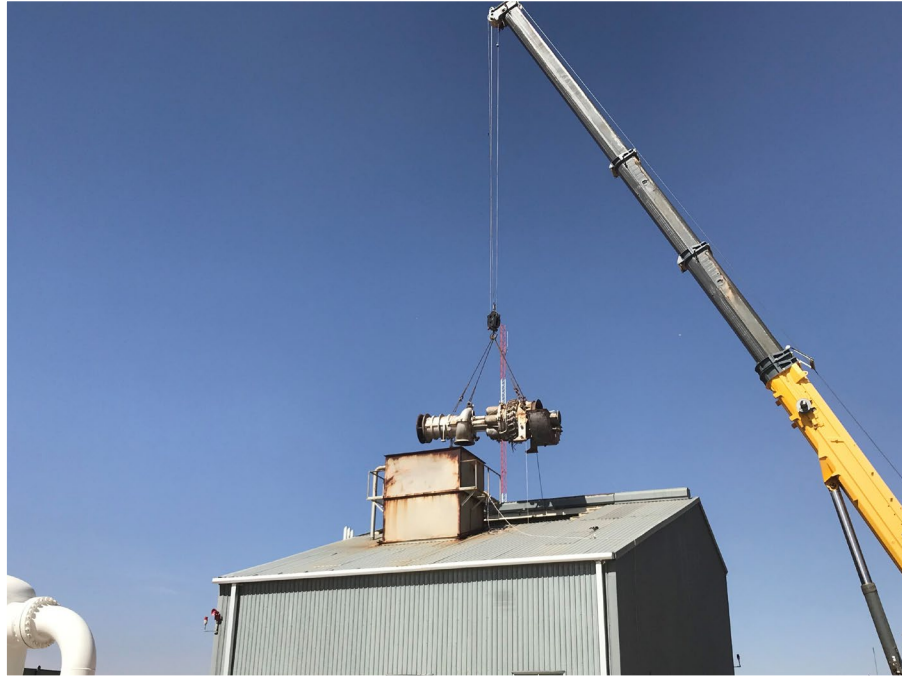
The original building was not constructed to accommodate turbine removal, so the unit had to be removed through the roof.
