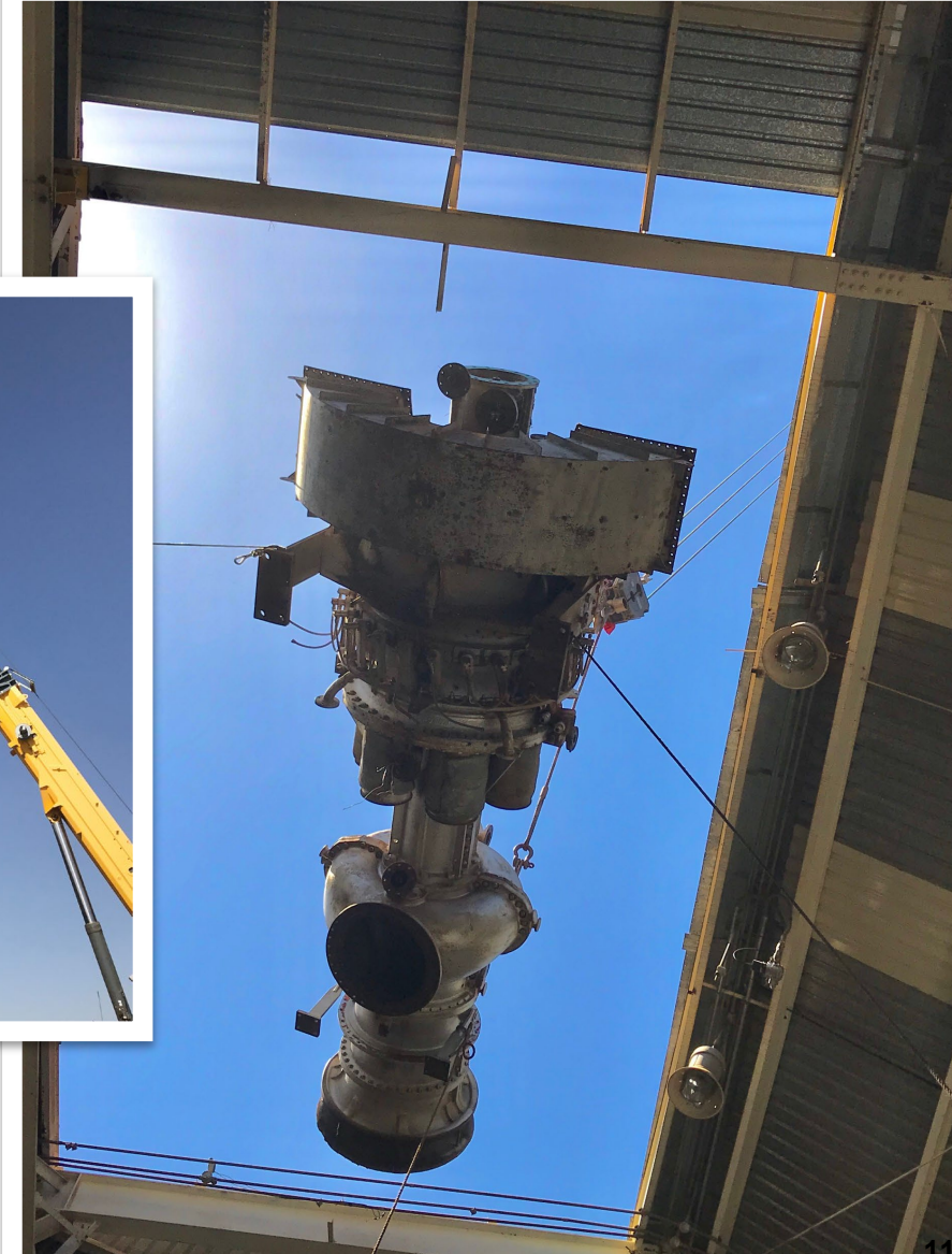
The original building was not constructed to accommodate turbine removal, so the unit had to be removed through the roof.
