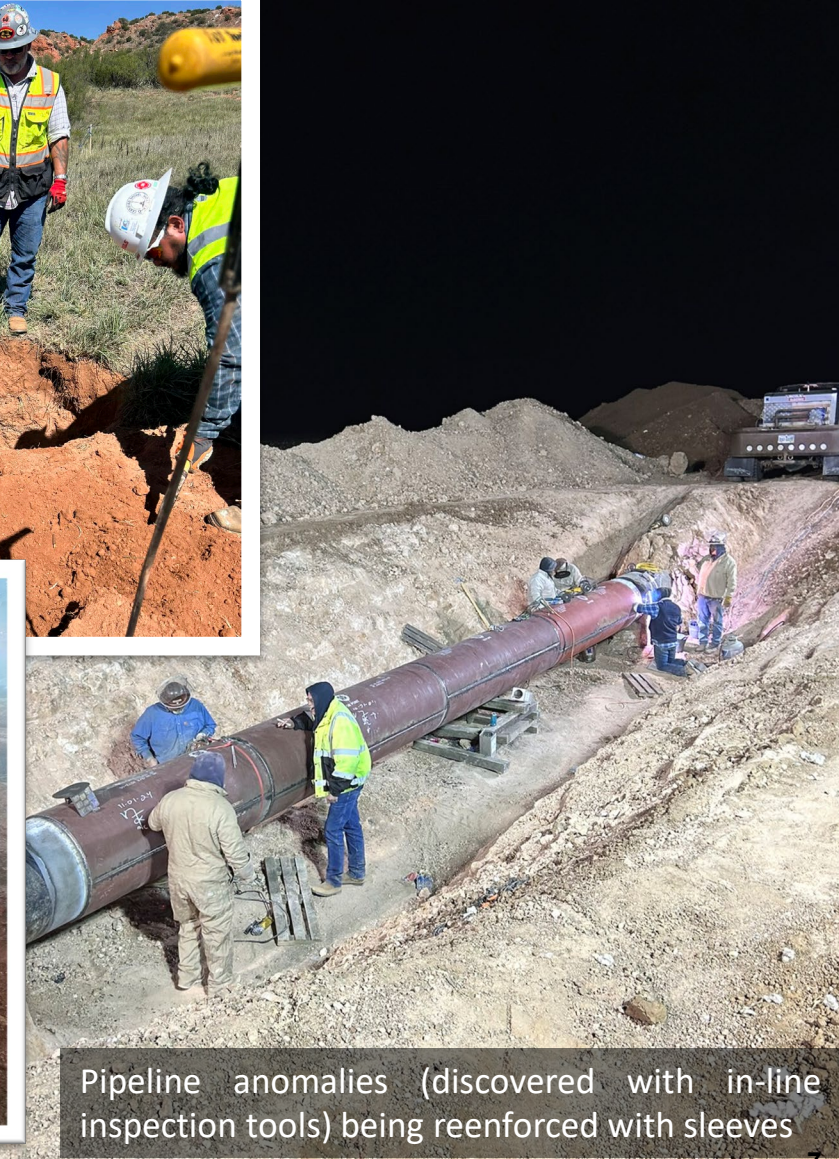
Excavation to evaluate anomalies and remediate pipeline damage as needed
