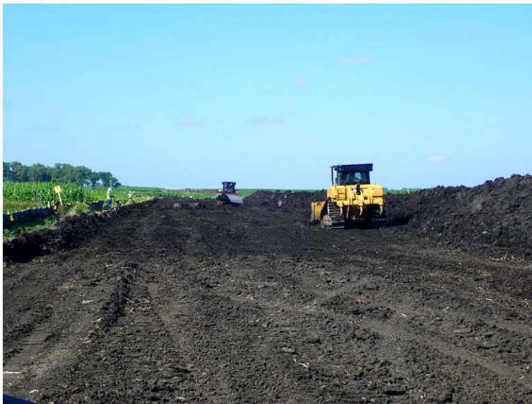
Facing southwest at MP 6.40, K & K removing and stockpiling topsoil
