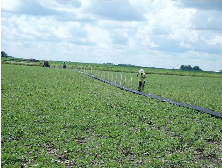
Facing northeast at MP 6.70, K & K installing ECDs
