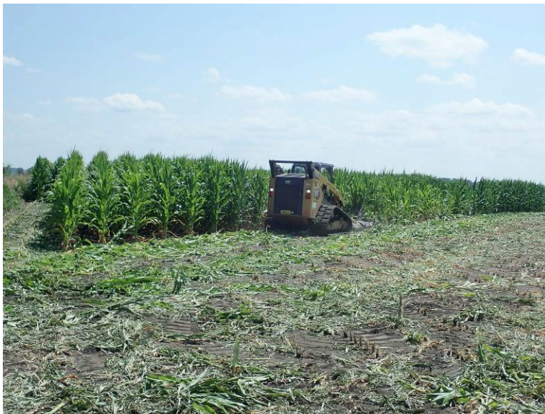
Facing southwest at MP 9.2, K & K mowing the ROW
