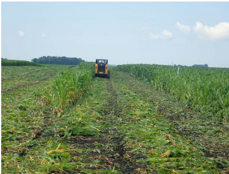
Facing southwest at MP 7.40, K & K mowing the ROW
