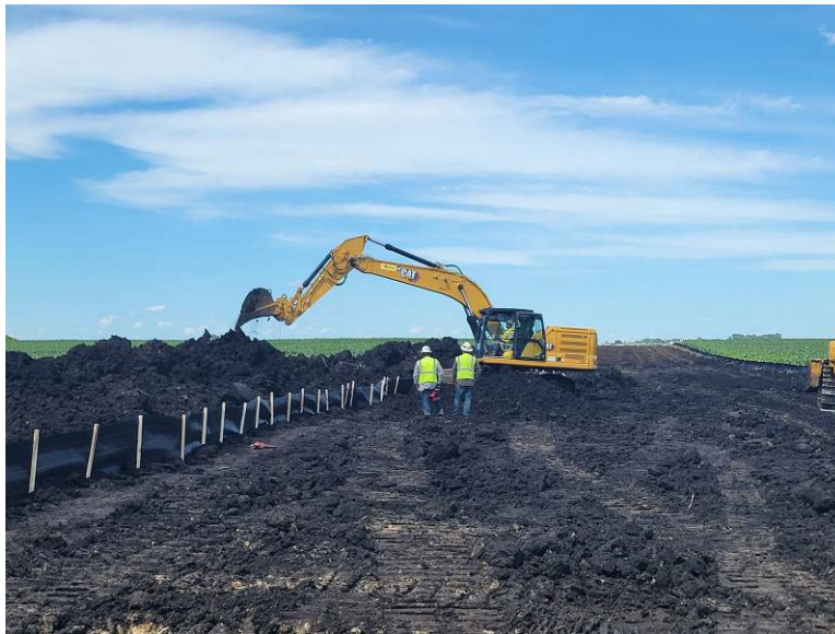
Facing southwest at MP 7.30, K & K removing and stockpiling topsoil
