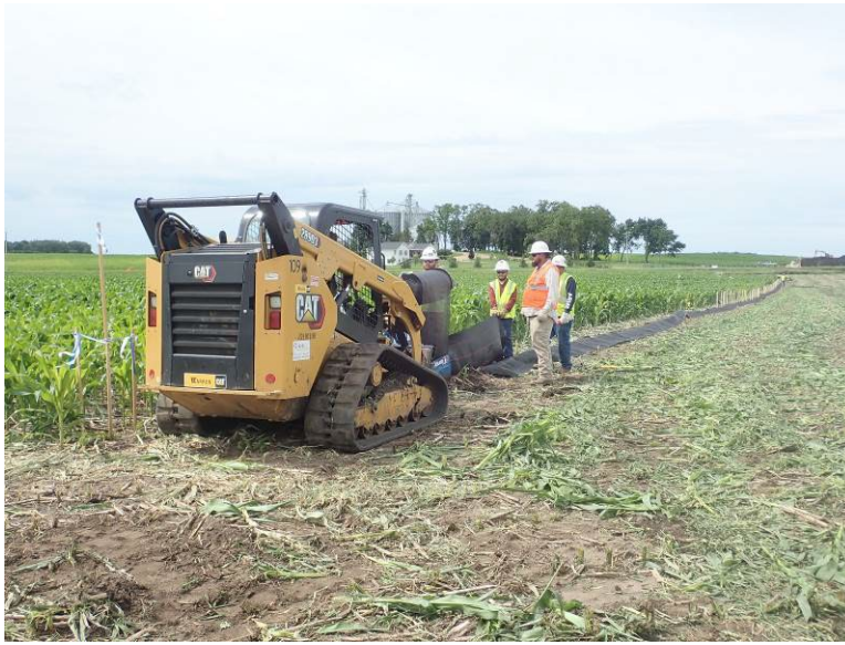
Facing southwest at MP 7.00, K & K installing ECDs
