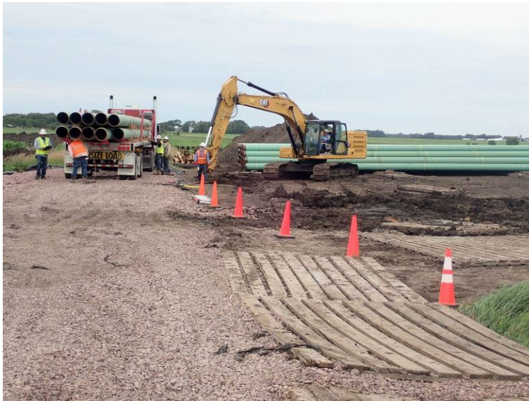
Facing northwest at MP 6.00, K & K offloading FBE piping
