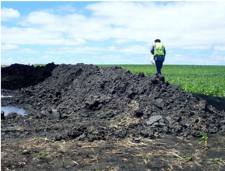
Facing southwest at MP 7.40, K & K seeding topsoil spoil piles with annual ryegrass for stabilization
