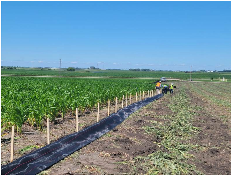
Facing northeast at MP 7.3, K & K installing ECDs
