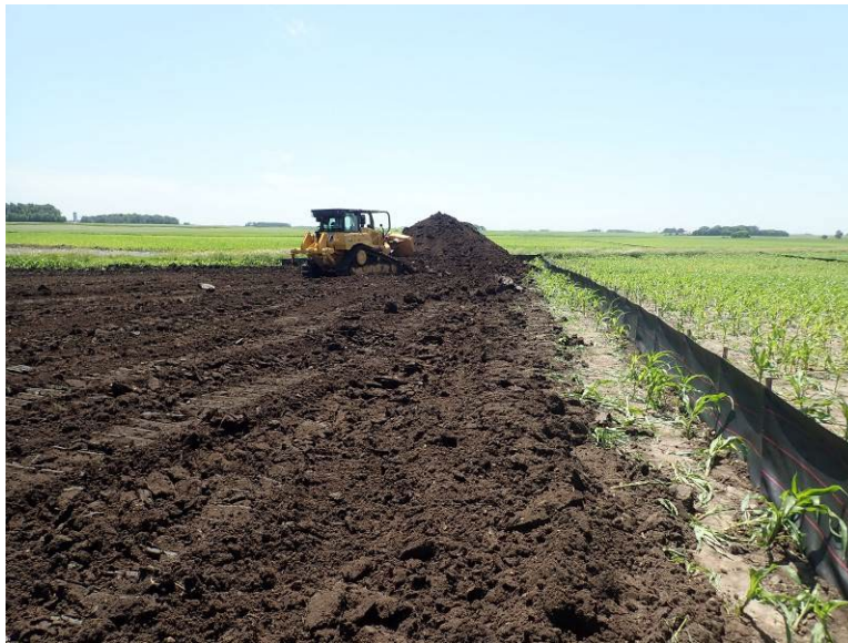
Facing southwest at MP 6.0, K & K removing and stockpiling topsoil
