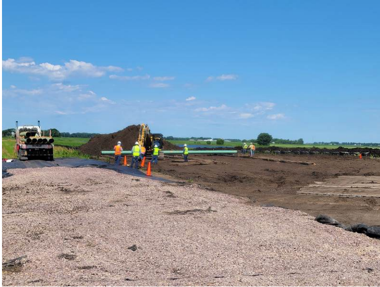
Facing northwest at MP 6.0, K & K offloading FBE piping
