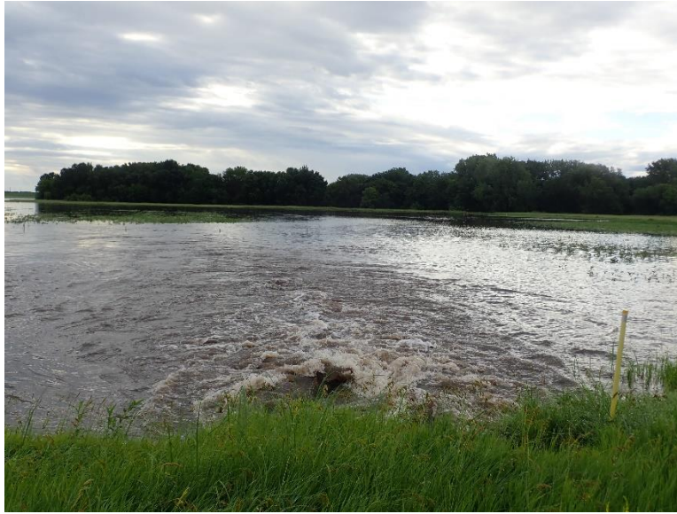
Facing northeast at MP 10.20, project area continues to be flooded due to excessive rainfall
