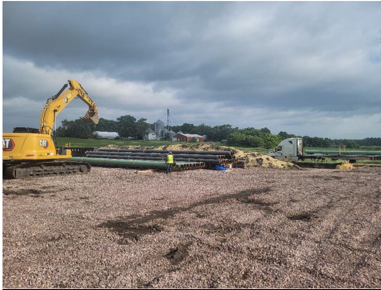
Facing north at MP 10.40, K & K offloading 16-inch-diameter piping
