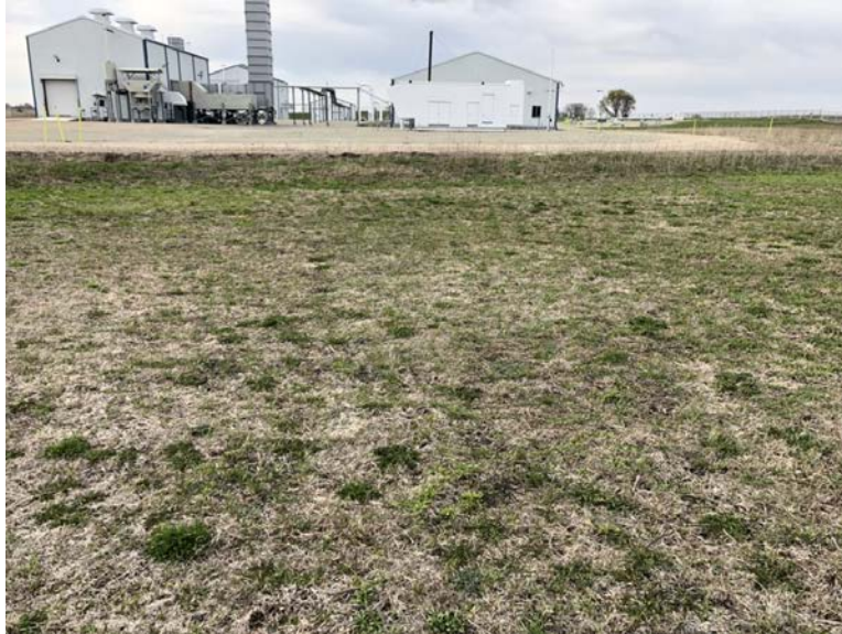
Facing south, view of north end of project
