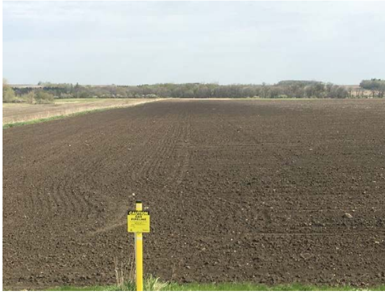
Facing north at MP 0.24, right of way reverted back to agriculture (corn), north of County Road 6 SW. Access road to HDD entry location for North Branch Root River, Wetland and County Road 108 SW
