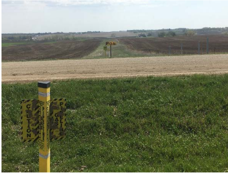
Facing west at MP 4.83, HDD location for 90th Avenue SW
