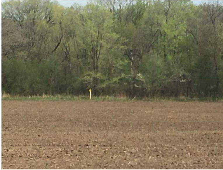
Facing north at MP 11.70, HDD entry location for Salem Creek (RGL-087-S1) and Wetland RGL-7-W1 north of private drive
