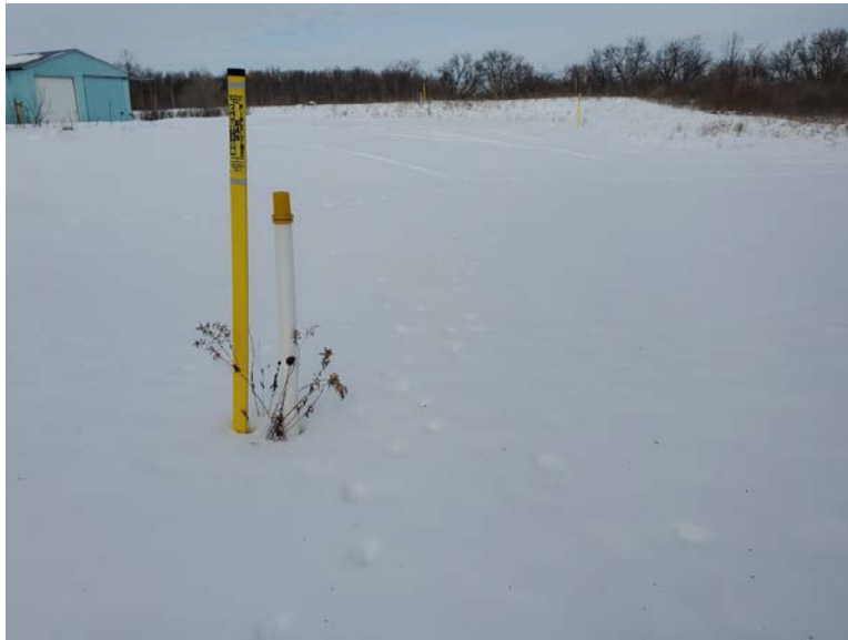
Facing northwest at the entrance to the Crow River HDD, site is snow covered and stable
