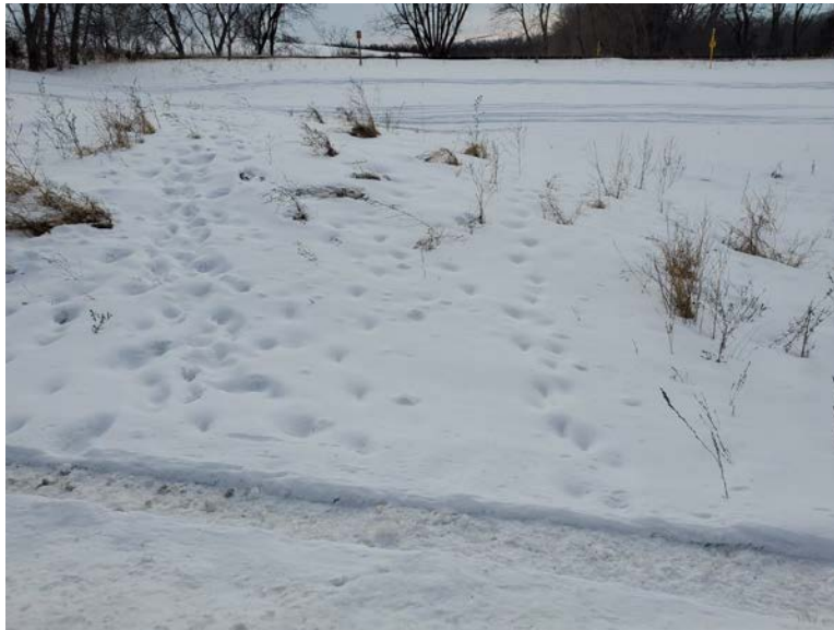
Facing south, erosion control blankets (ECBs) in roadside ditch, temporary access road south of 37th Street, site is snow covered and stable
