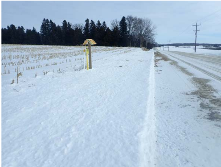
Facing west at MP 6.45, ECBs and repaired ruts are snow covered and stable.
