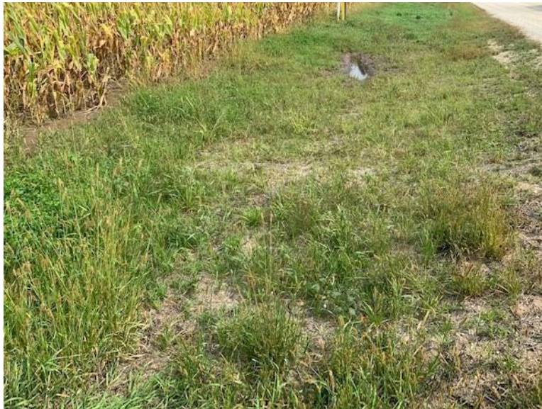
Facing east at MP 6.45, ECBs and vegetation impacted by landowner's tractor tires
