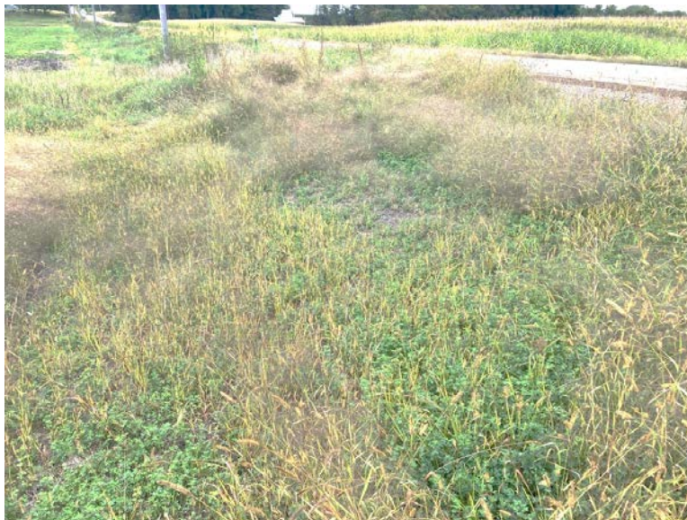
Facing east near MP 0.1, north side of 134th Street, erosion control blankets (ECBs) in roadside ditch, 70% vegetative coverage
