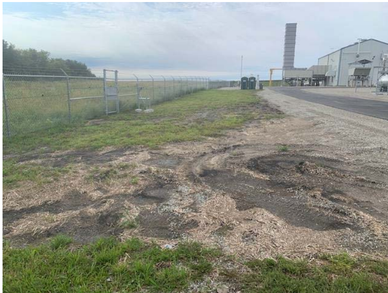
Facing south, environmental inspector reseeded and mulched the former office trailer location September 21, 2020, 50% vegetative coverage
