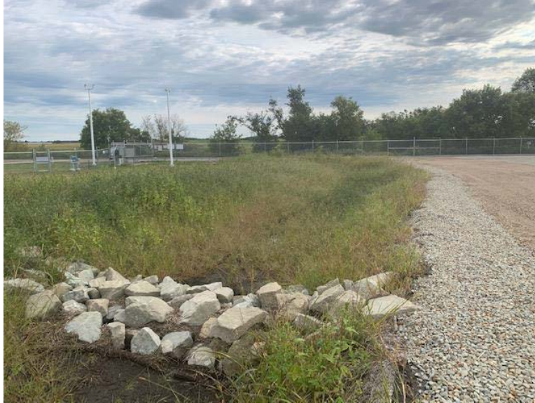
Facing west, infiltration trench at 65% vegetative coverage
