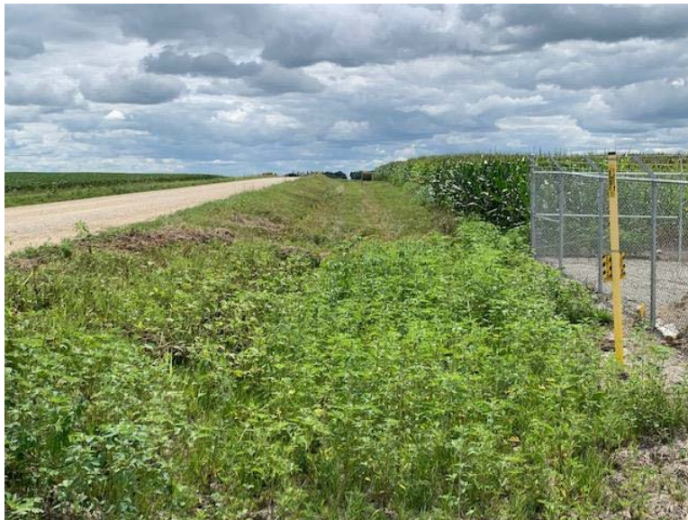
Facing south, ECBs in roadside ditch west of 560th Avenue, vegetation has reached 70%
