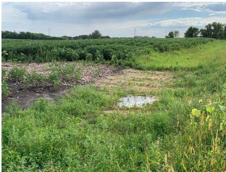
Facing east at MP 7.44, ECBs in roadside ditch north of Division Street East
