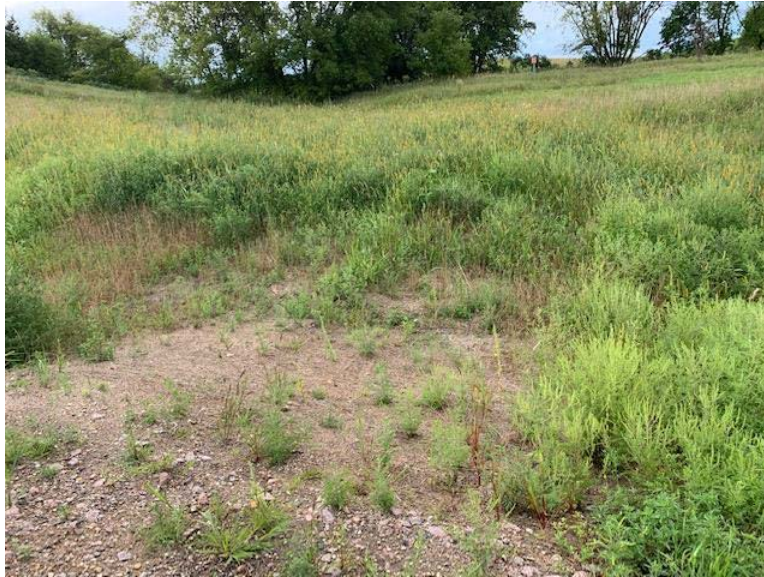
Facing south at MP 1.35, ECBs in roadside ditch south of 37th Street Southeast, vegetation has reached 10%
