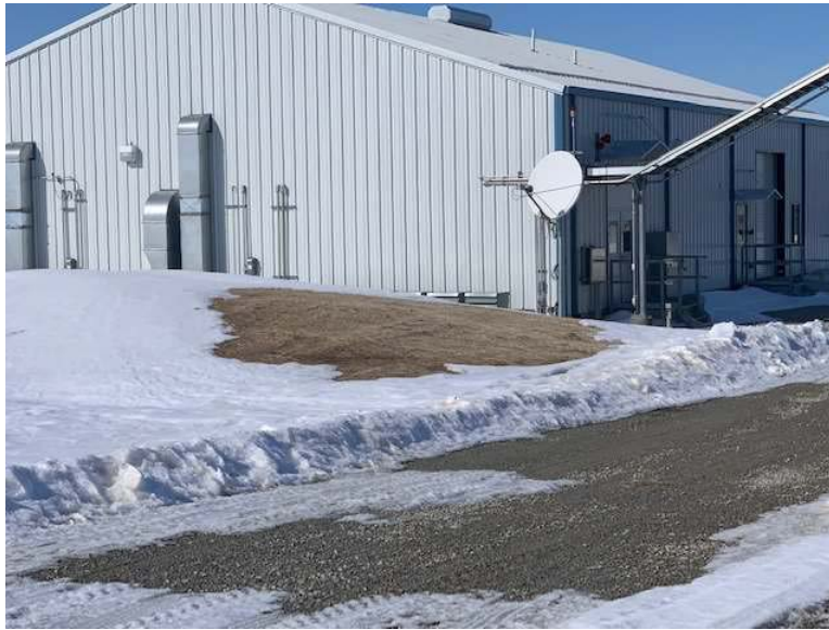
Facing northwest, erosion control blankets covering the septic mound south of the auxiliary building
