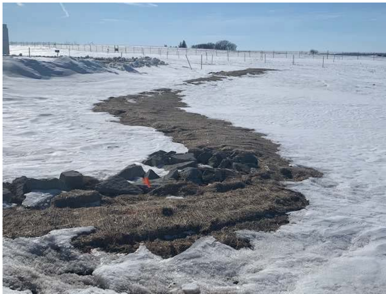
Facing west, Erosion control blankets covering infiltration trench north berm
