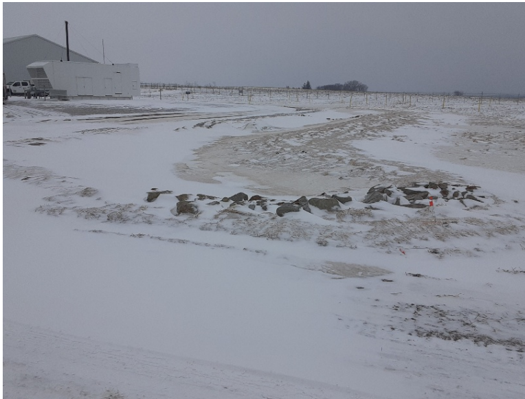
Facing southwest, erosion control blankets along berm of infiltration trench
