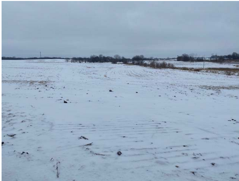
Facing east at MP 1.7 access road, erosion control blanket is in good working condition
