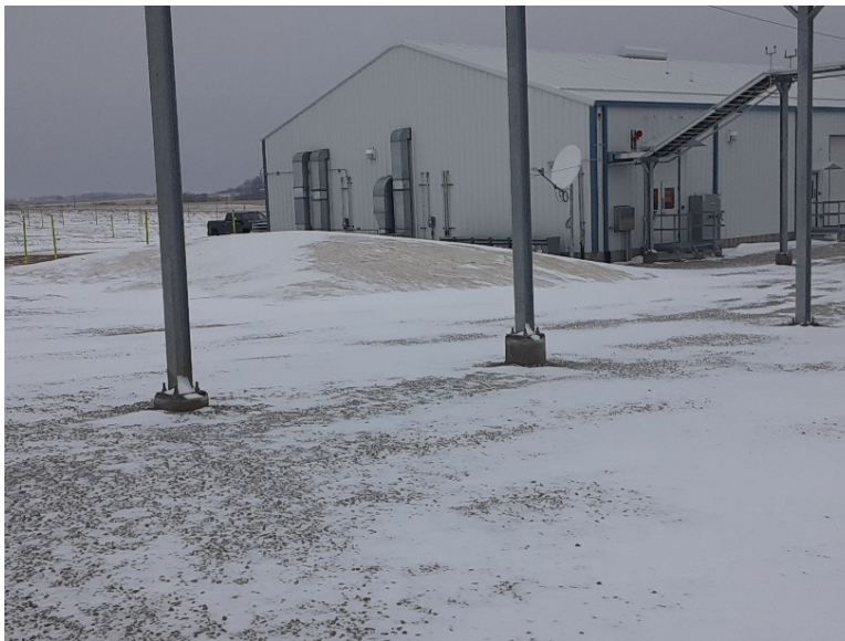
Facing northwest, erosion control blankets for the septic system mound
