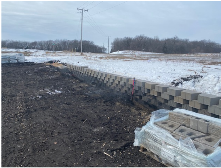
Facing west at MP 0.0, Minnesota Limited constructing retention wall
