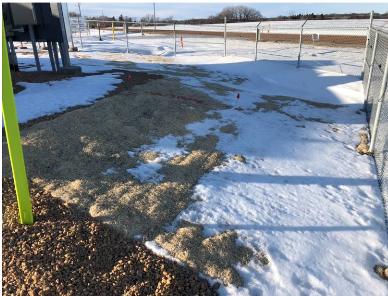
Facing west, view of the northwest corner of the compressor station
