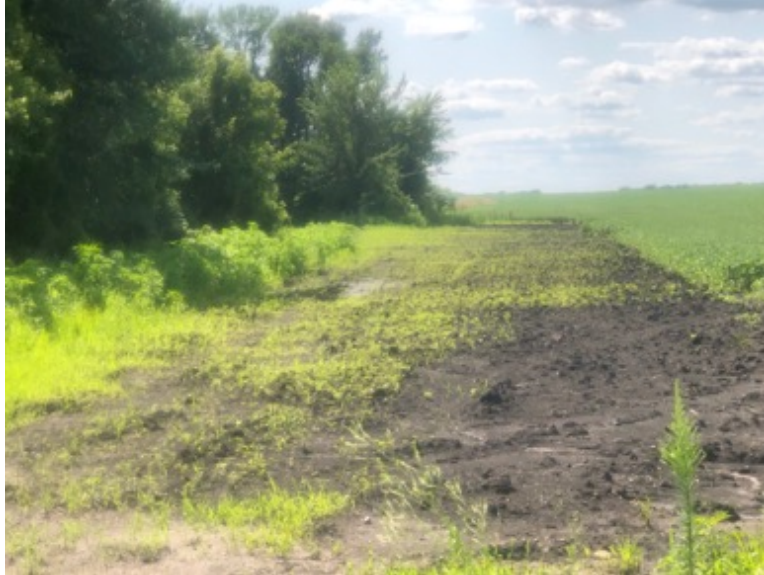
Facing west at MP 0.45, temporary access road west of CR-143 returned to agriculture; native grasses are coming in voluntarily
