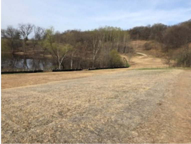
Facing southwest, MP 3.0 to MP 3.1, redundant silt fence around Buck Pond, Shannon Montante (Dakota County Parks) has accepted responsibility for maintenance and eventual removal of this fencing. Dakota County is providing their own restoration of this park area.
