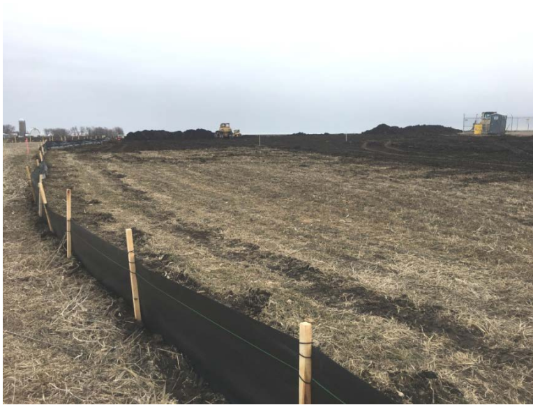
Facing north, commenced installation of silt fence and erosion control devices
