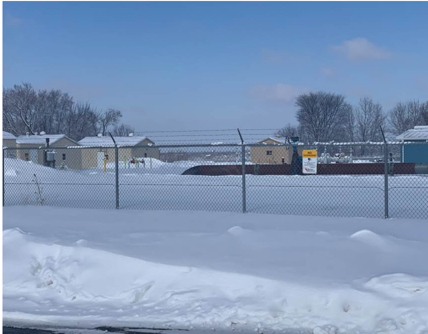
Facing northwest at MP 7.8, Cedar Station launcher/receiver
