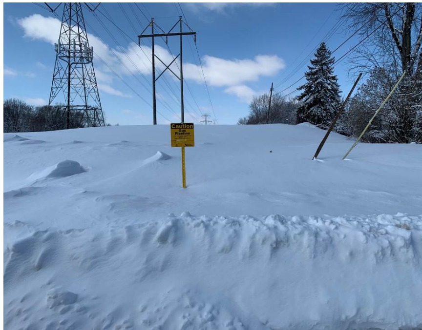
Facing west at MP 6.5, R.O.W. west of Sandstone Drive
