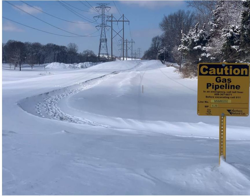
Facing east at MP 6.26, ROW and extra temporary workspace east of Rahn Road Walking Trail
