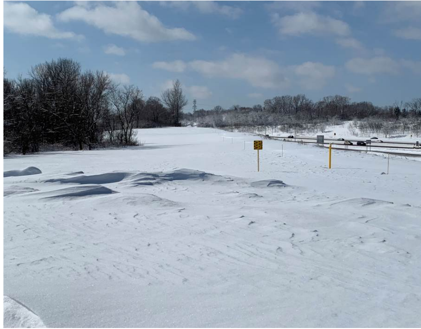
Facing southwest at MP 7.4, extra temporary workspace southwest of Diffley Road
