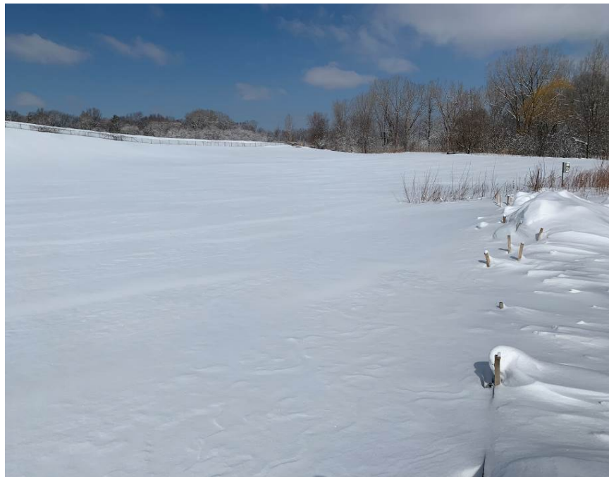
Facing northwest at MP 7.0, extra temporary workspace and silt fence covered by snow west of Nichols Road
