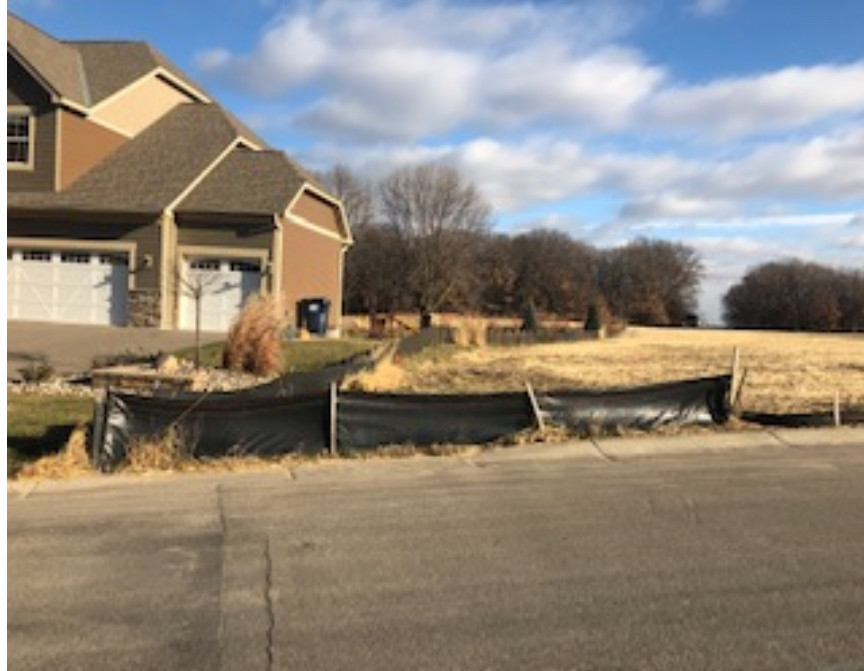
Facing east, MP 3.3 Interlachen Dr., inspection found no erosion
