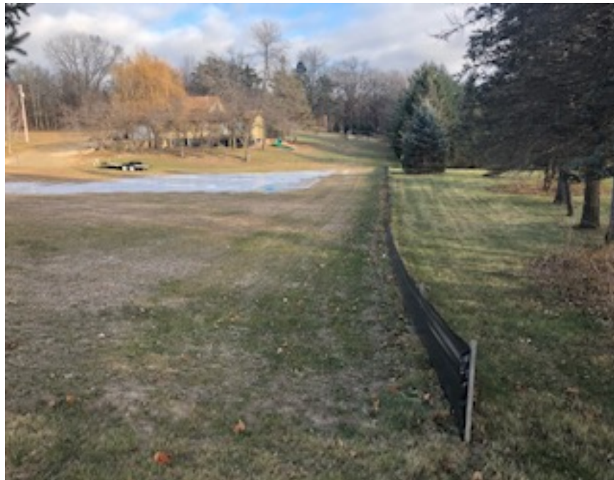
Facing east, MP 1.0, S. Roberts Trail, inspection found no erosion
