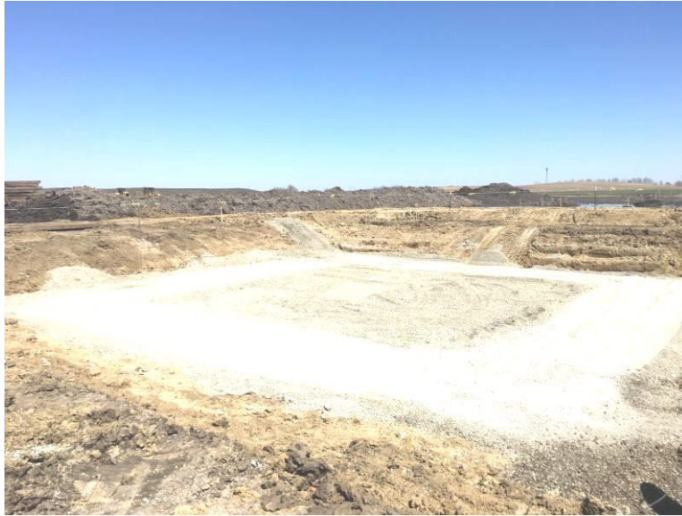
Facing northeast, commenced excavation for the auxiliary building foundation
