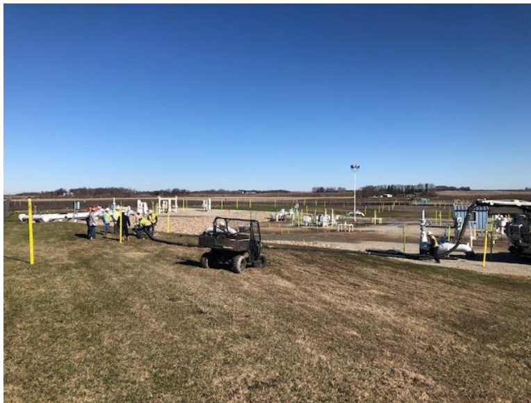
Facing north, contractor commenced hydro-excavation of the MNM 80102 (B-line suction)
