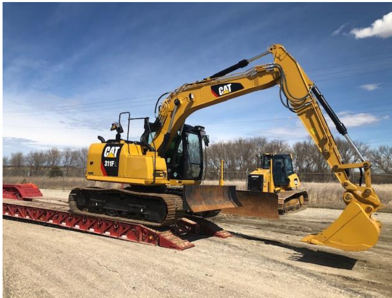
Facing northeast, contractor offloading a tracked excavator
