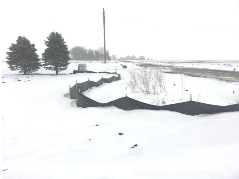
Facing south, silt fence is functional and in good condition, the project received approximately 12 inches of snow April 10-12, 2019
