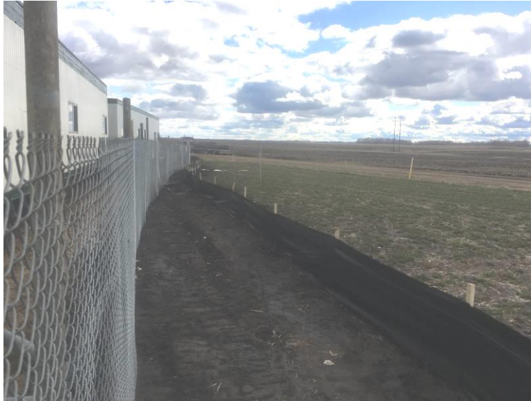
Facing south, silt fence is functional and in good condition
